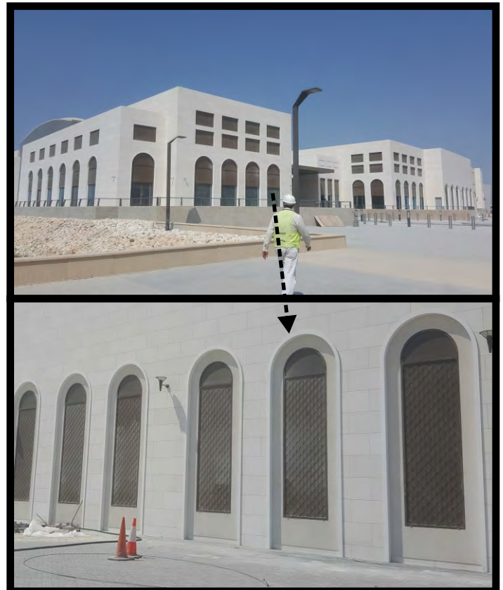
VORACO Scope of Work: GRC 6M Architraves. Project : THE AVANUE MALL
